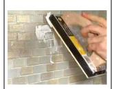
While the grout is still fresh, stroke diagonally the long edge of the grout float to remove excess grout and then wipe it with wet sponge to clean.
